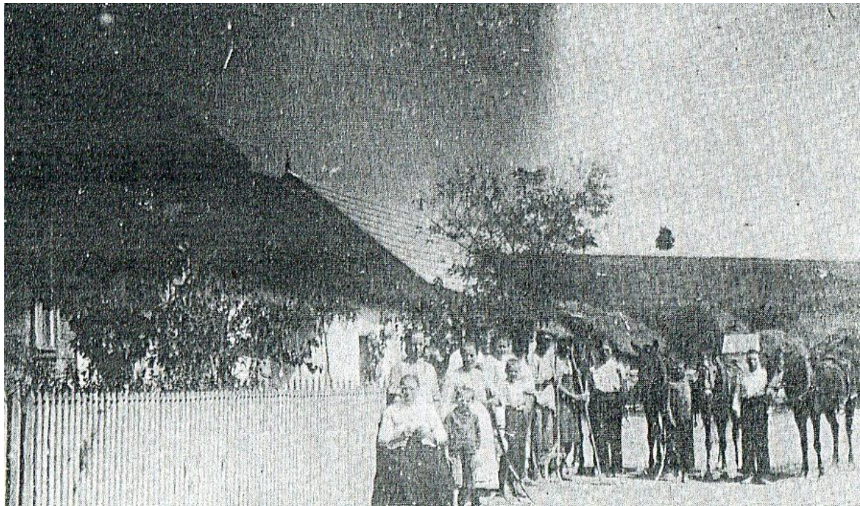
On the Farmyard of Reinhold Suckut (Lower Village) in August 1940
