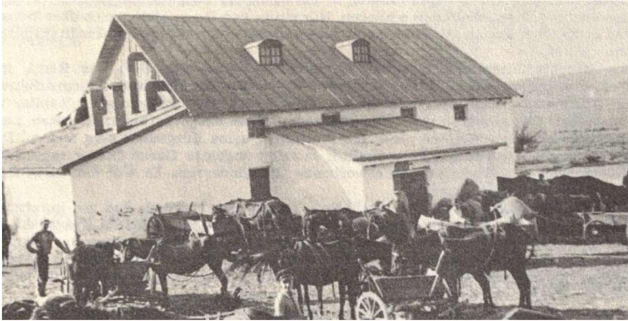
Karl Wildermuth's Mill in Nikolajewka, built in 1919 by Jakob Wildermuth. In 1934, the operation was fundamentally modernized. With the installation of four double roller mills and other modern machines, the daily output could be improved to fifteen tons [1 ton = 1,000 kilograms or 2,205 pounds]. The attached oil mill achieved a daily capacity of seven tons.
