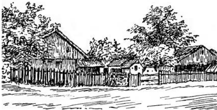
Enclosed Yard in Atmagea
